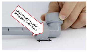
Push the pipe firmly into the fitting until the end reaches the line marked by the felt-tin pen. Thus, with a quick look we check that it is properly joined.
