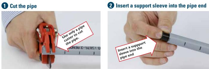
Use only a pipe cutter to cut the pipe. Never use a hacksaw. To ensure a clean, square cut, rotate the pipe whilst maintaining pressure on the cutter until the pipe is severed.
