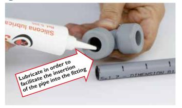
The outside of the pipe or the inside of the fitting (specially the grab ring) shall be lightly cleaned and lubricated in order to facilitate the insertion of the pipe into the fitting.
